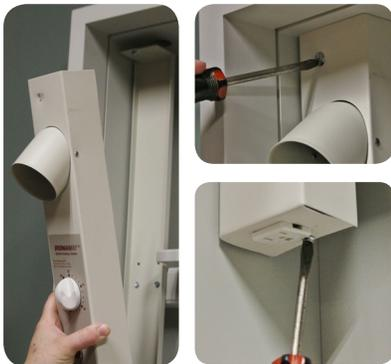
Return raceway to unit, screwing top and bottom screws to hold in place.
