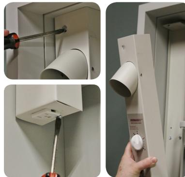
Begin removing electrical raceway from unit by removing small screws at the top and bottom of raceway with a flathead screwdriver. Gently pull raceway out of unit, being careful of wires that are still connected.
