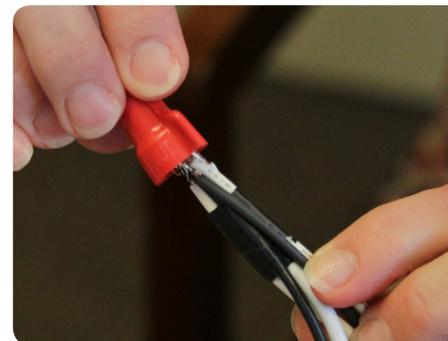
Locate dark grey wire at back of timer and lay it flush with striped ends of white wire bundle. Replace wire nut by screwing clockwise with downward pressure. **Note: make sure wires are snug and cap is secured tightly.**
